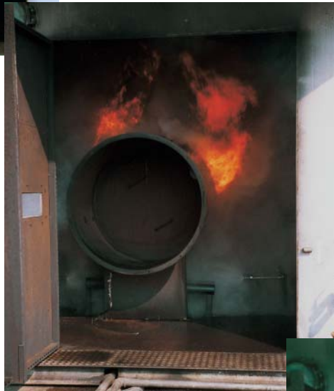
Instant dampening of the flames on actuation of the AquaSafe system
